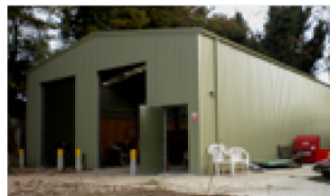
10m x 20m Machinery store
