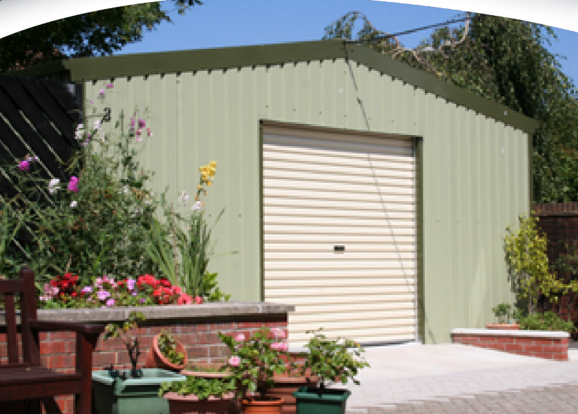
8m x 6m Storage building
