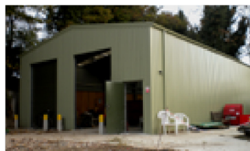
10m x 20m Machinery store
